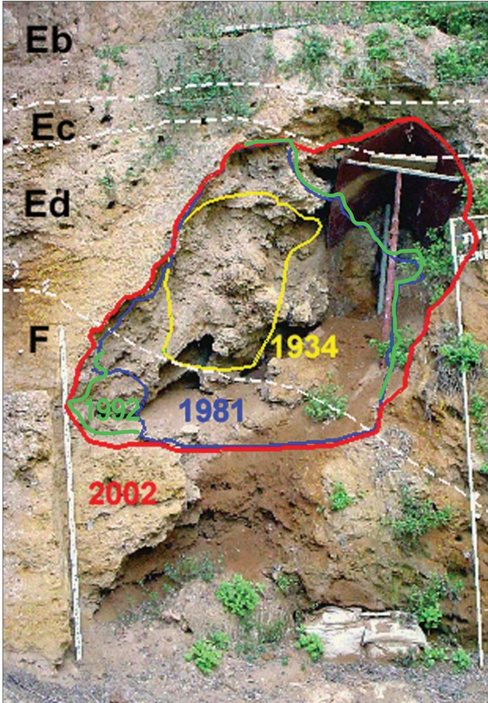
Figure 7: The changing contours of the cavity's mouth 1934-2002.
